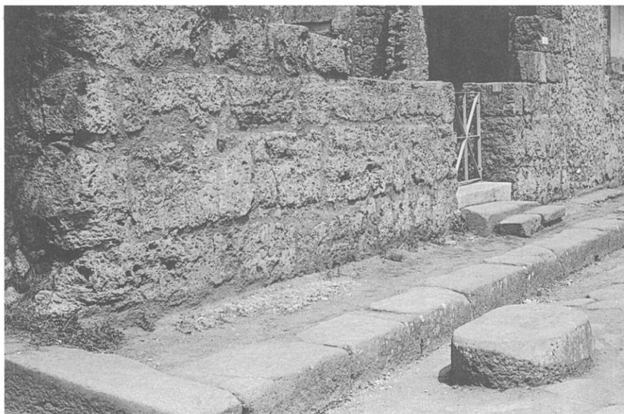
Fig. 1. Tufa blocks extensively used in house construction within the Roman town of Pompeii, Italy.
