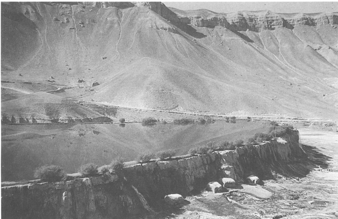
Fig. 28. The massive but thin-walled barrage and lake at Band-e-Amir, Afghanistan (photo by W.E. Renshaw).
